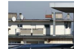
Power cable on the roof
