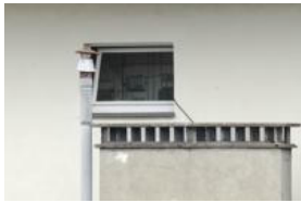
Power cable reaching the socket
