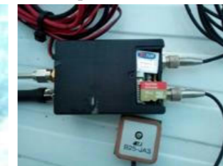
Inside the thingy with antennas and cards (below with a brown outline is the GPS)
