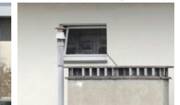
Power cable reaching the socket
