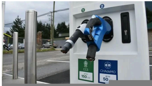
Electric vehicle charging station with severed cables.
