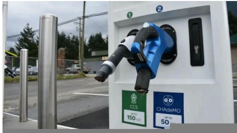
Electric vehicle charging station with severed cables.
