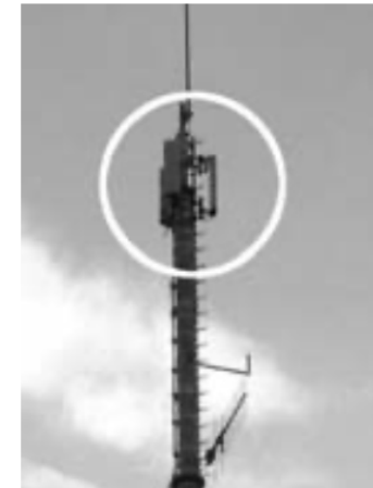
TETRA antenna (very similar to cellphone antennas; three antennas are a characteristic feature).
