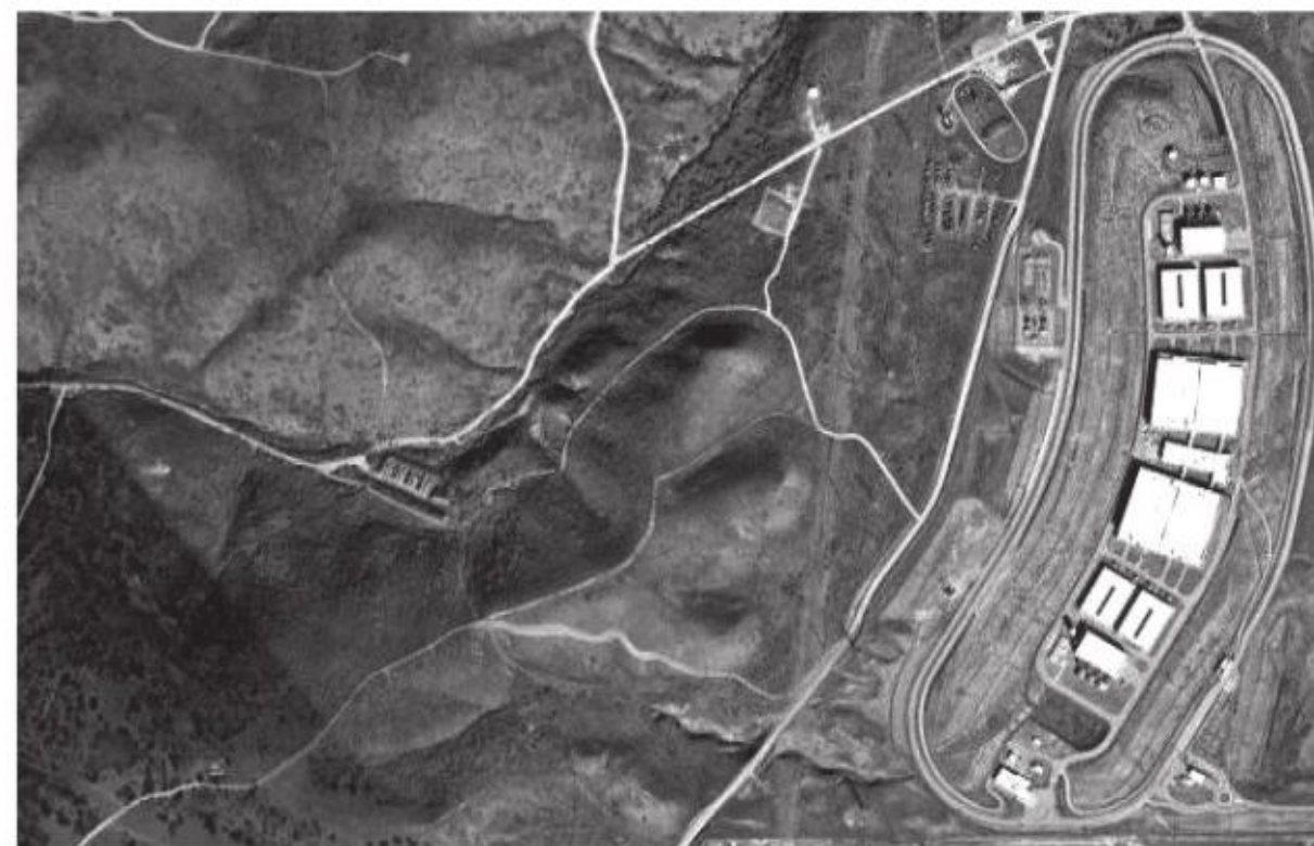
Intelligence Community Comprehensive National Initiative Data Center in Utah
